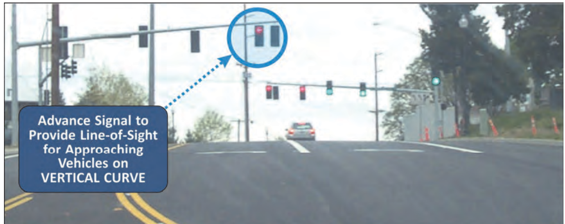
Exhibit 4-13 Advance Signal Placement to Address Vertical Curve
