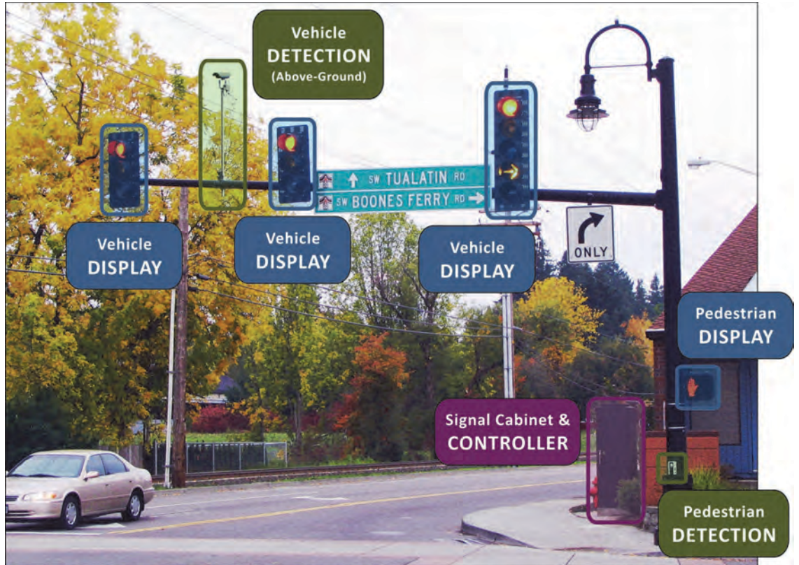
Exhibit 3-2 Common Signalized Intersection Components
